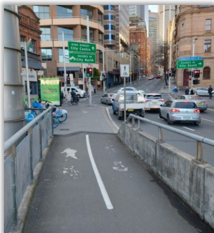
Photo 4. Shared path in Darling Harbour (photo: John Sergeant)
