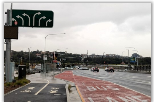
Intersection of Victoria Road & City West Link, Rozelle Interchange (Photo: V. Simpson-Young)
