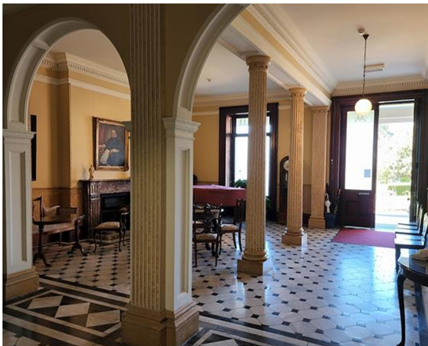
The front hall of Toxteth Park was created in the 1880s by demolishing two walls of Verge's parlour and introducing pilasters, archways, a painted dado and a marble floor (Image: Ian Stephenson)
