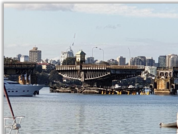
Glebe Island Bridge – note the yellow buoys placed to protect the crumbling timber from further damage (photo: V. Simpson-Young)
