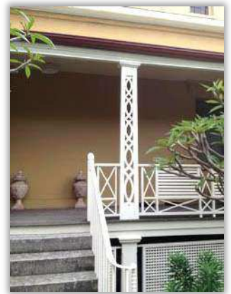
Picture 2: New timber fretwork infills installed in 2016 (image: Robert Hannan)
