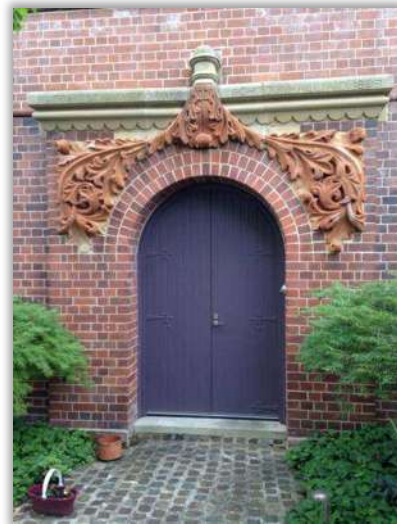
Former Methodist Church Hall, Toxteth Rd (1898). Note the cartouche and the acanthus trails rendered in sandstone which give the entrance a certain grandeur and éclat. (image : Martin Lawrence)
