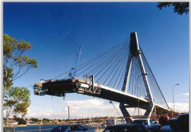
The Anzac Bridge under construction (image: John Symonds)
