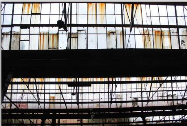
Sawtooth roof of the Tramsheds (image: Jodeska)
