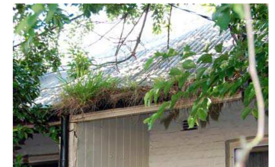
Weeds growing in the gutter of a house in Westmoreland Street. Photo: Bruce Davis
