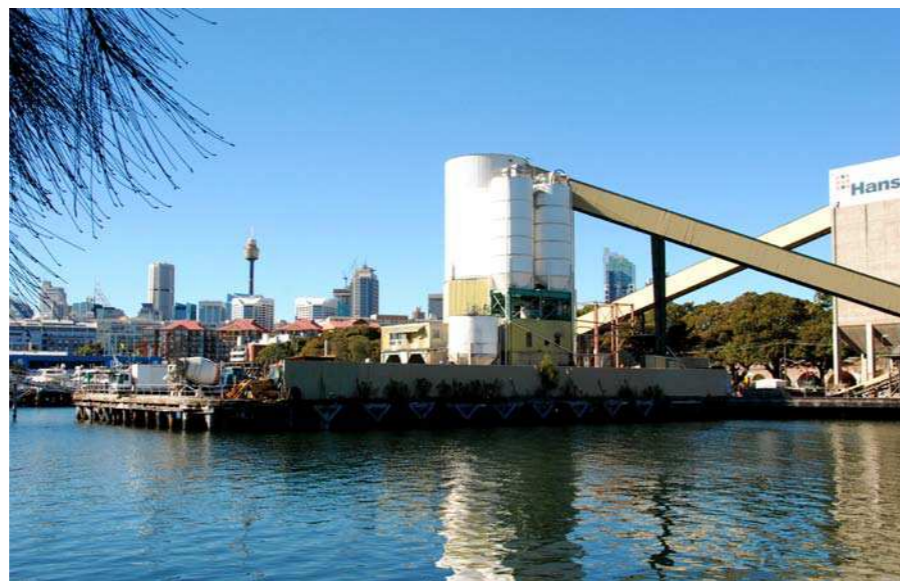
Will the Hansons concrete batch plant move from Blackwattle Bay to Glebe Island? Photo: Bruce Davis
