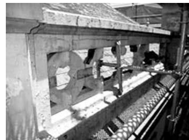
Deteriorated parapet
