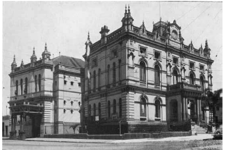
View of Glebe Town Hall showing the portico to Mt Vernon Street, now demolished. From the 1935 City of Sydney Annual Report
