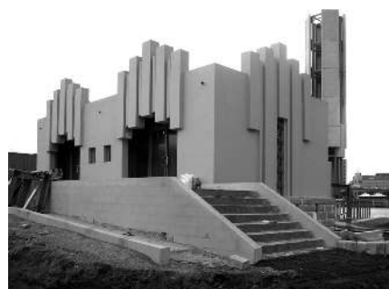
Burley Griffin Incinerator. Photo: Davis Mander Jones
