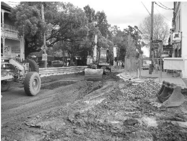
Work in progress, Glebe Point Road, August 2008.
