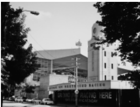
The now-demolished entrance plaza seen from Wentworth Park Road.
