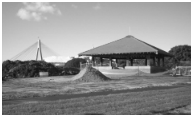
The Pavilion, surrounded by park restoration work. Photo: Edwina Doe
