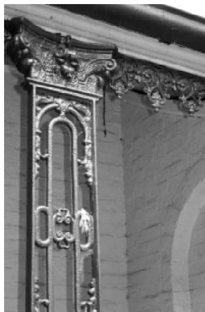
Laurel Tree House , Arundel Street: detail of a cast iron grille column, complete with an elegant capital. Photo: Bruce Davis
