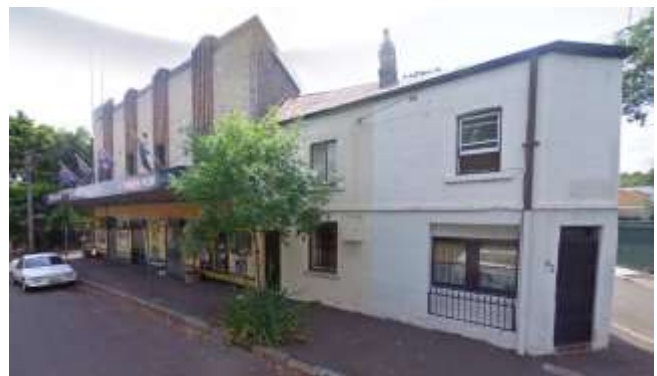
Figure 2 The hotel(left of image). It occupies a small site and is in close proximity to houses (right of image)
