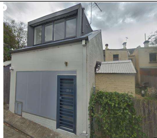
Figure 2 In 2016 approval was given to convert the garage into a two storey house
