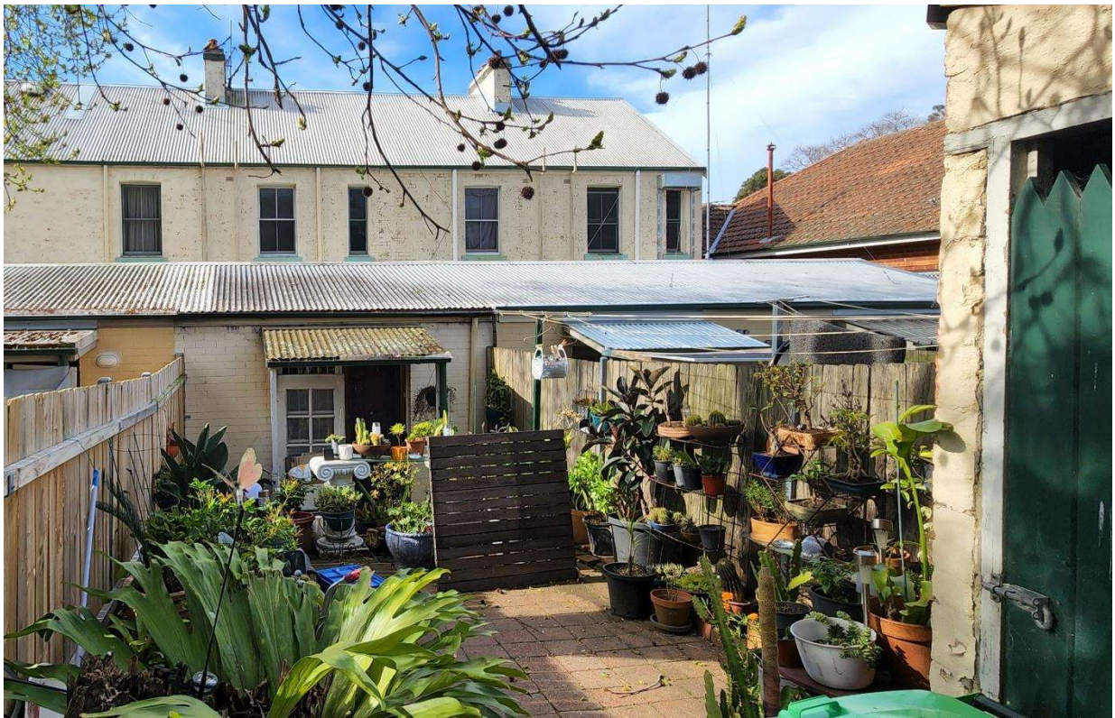
Figure 10 In the 1980s the NSW Inner City Housing Team added a shallow roofed single storey service wing to the rear of a row of terrace houses at 36-44 Campbell Street. It is seen here from Campbell Lane. In Denman Lane a small low building built on the lane frontage and retaining the outhouse could be compatible with the heritage conservation area and be a model for any further rear lane development in the row.
