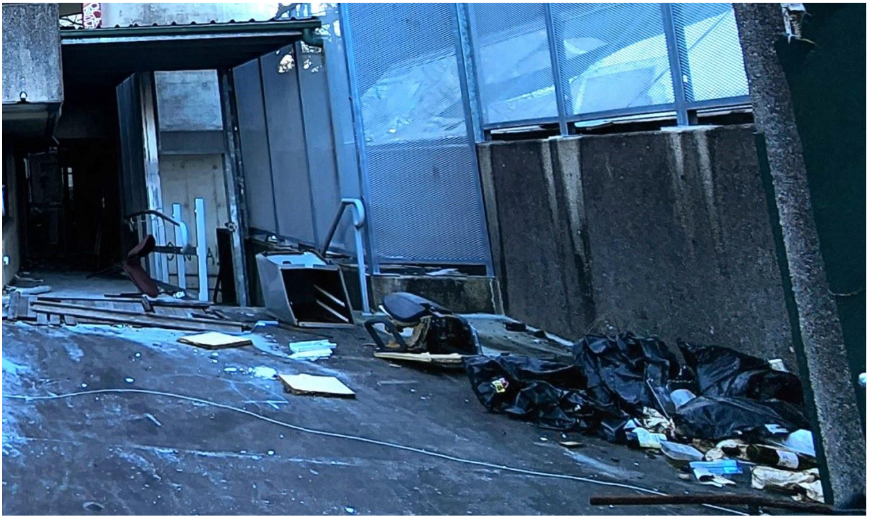
Figure 4 The area between Bidura and the former Metropolitan Remand Centre is littered with rubbish and is a haven for vermin
