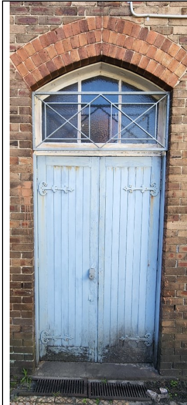
Figure 2 Door D2 is an original door which retains its elaborate Gothic revival hinges. The transom window above is also original
