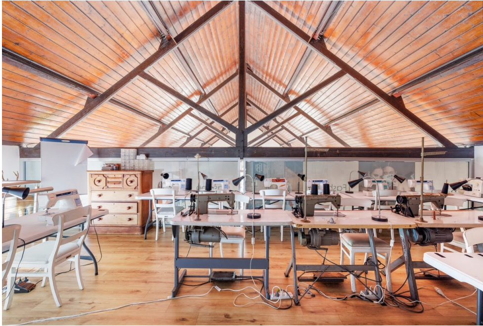
Figure 6 The roof in the existing mezzanine
