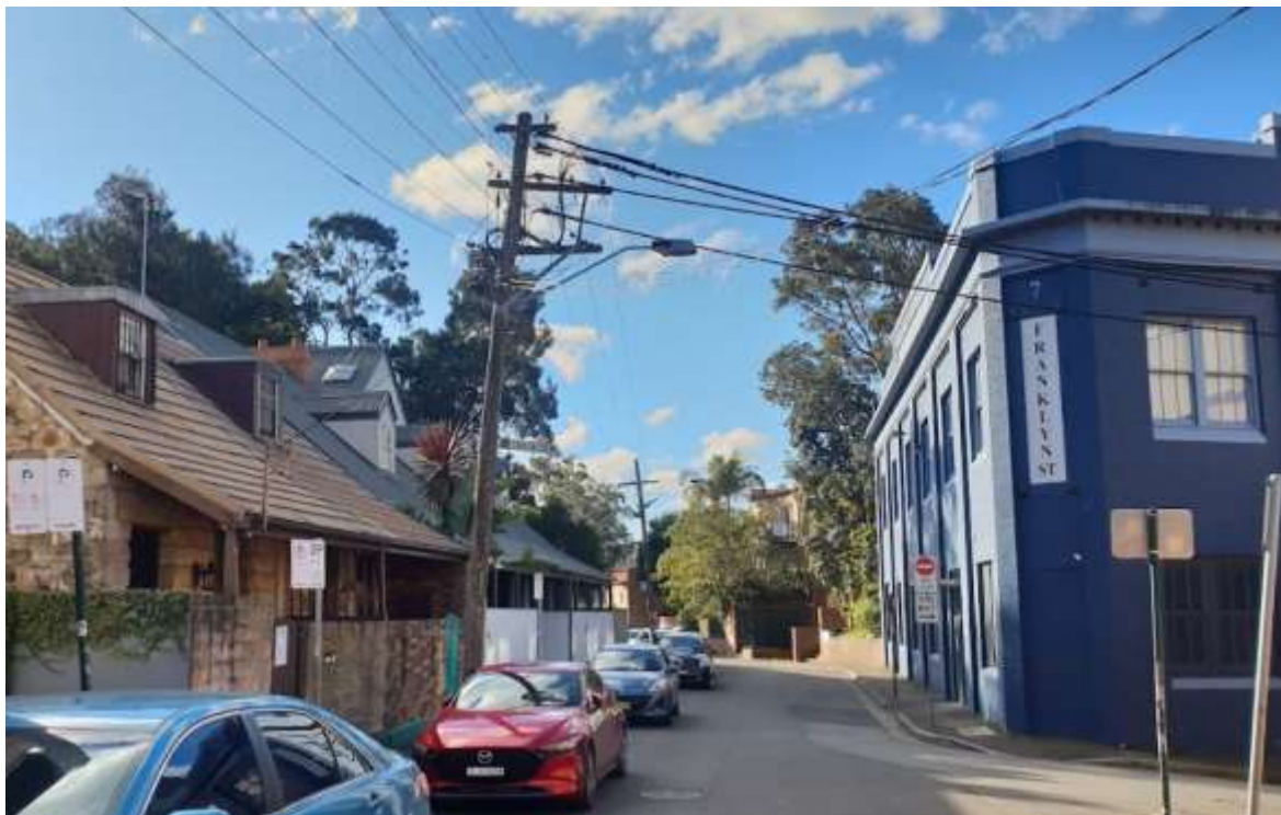
Figure 1 The proposal involves demolishing the warehouse shown on the right and its neighbour, not pictured, in Greek Street. Number 7 Franklyn Street makes a significant contribution to the streetscape and the character of the area.
