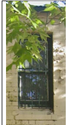
Figure 7 The window which is to be relocated
