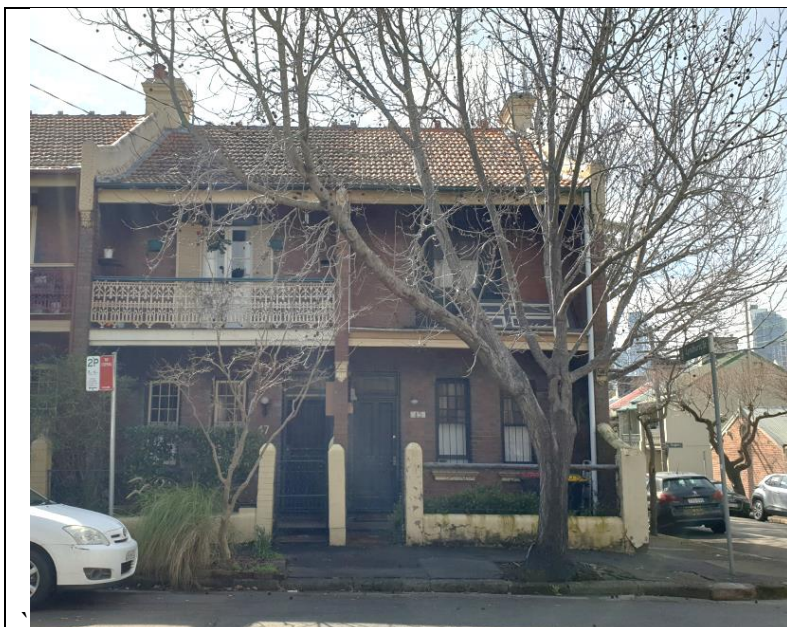
Figure 1 Numbers 45 and 47 Darghan Street are a matching pair of houses. The attic addition which has been approved for number 45 does not include a dormer on the front elevation
