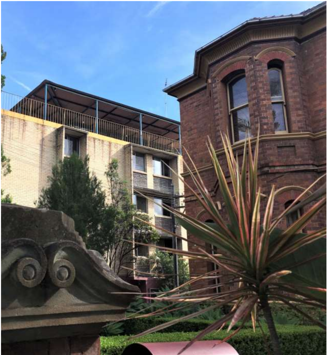
The roof terrace at 262-264 Glebe Point Road viewed from the neighbouring house at 266 Glebe Point Road.
