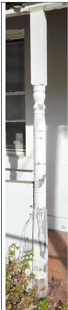
Figure 98 One of the verandah columns
