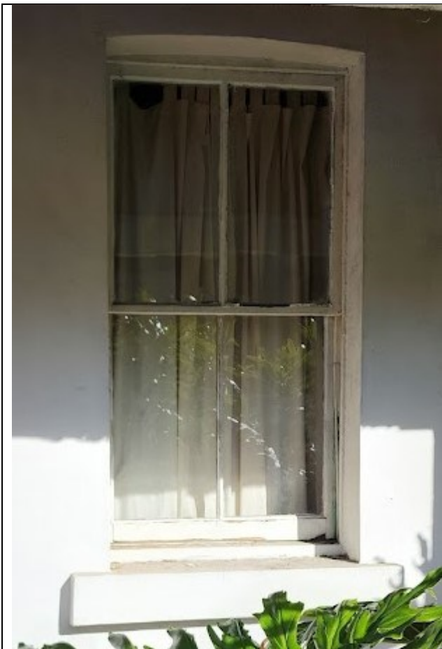
Figure 11 One of the three sash windows on the eastern elevation
