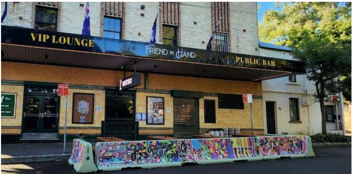
Figure 1 The outdoor dining area is close to many houses, particularly numbers 60 and 62 Cowper Street whose living rooms and bedrooms have no setback from the street.
