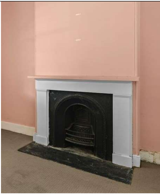
Fig 6, 7: the chimney piece, staff moulds, chimney and chimney pots and palisade fence (see Figure 9) are typical of a house dating from the middle of the 19 th century
