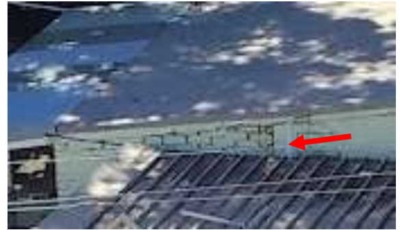
Figure 25 The skillion wall on the western side of the house was built in two stages. The brickwork of the northern end was not tied into the earlier wall. The crack relates to the method of construction rather than subsidence
