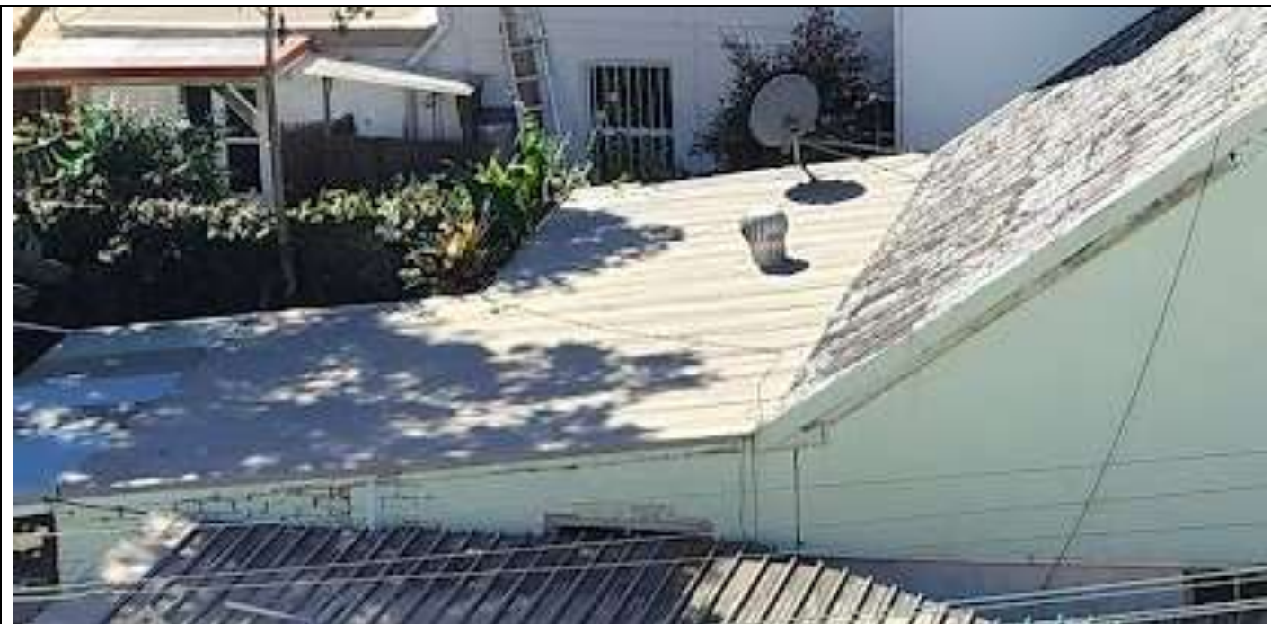
Figure 18 The western elevation of the rear skillion
