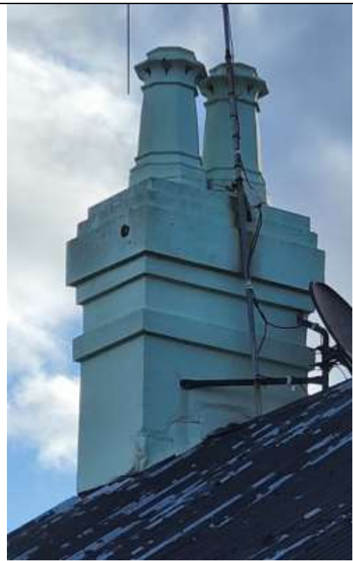
Fig 6, 7: the chimney piece, staff moulds, chimney and chimney pots and palisade fence (see Figure 9) are typical of a house dating from the middle of the 19 th century
