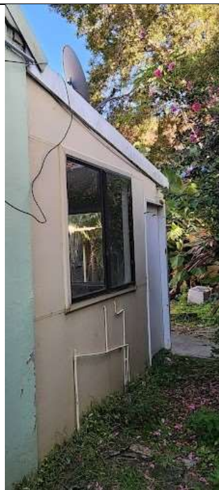
Figure 19 The eastern elevation of the rear skillion
