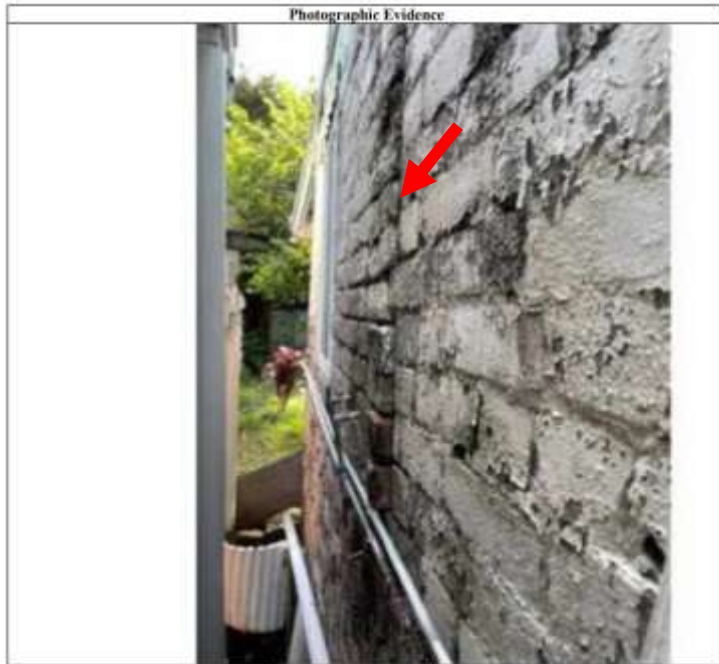
Figure 25 The skillion wall on the western side of the house was built in two stages. The brickwork of the northern end was not tied into the earlier wall. The crack relates to the method of construction rather than subsidence
