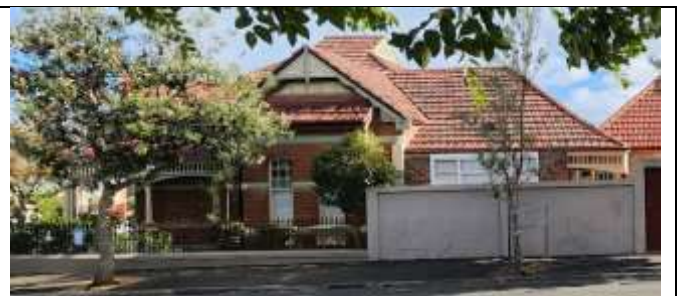
Figure 4 The existing boundary wall on the Maxwell Street verandah is obtrusive
