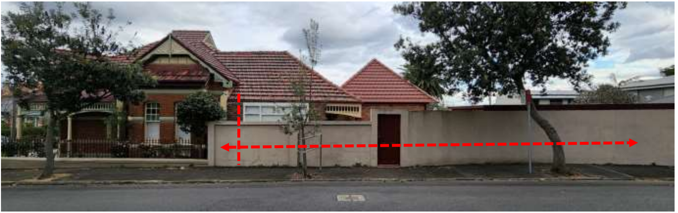
Figure 2 The brick wall on the Maxwell Road frontage is obtrusive
