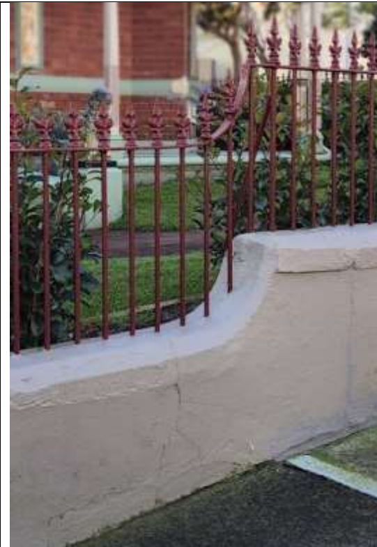
Figure 6 The original fence of 43 Toxteth Road shows the traditional way in which changes of height were transitioned and how the top of the masonry fence was defined with a capping
