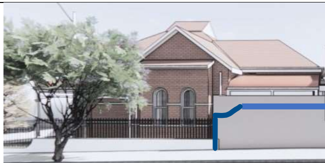
Figure 9 The fence should be redesigned using the principles of the NSW Heritage Office's Design in Context referred to above. It should be lower, transition in height and have a capping.
