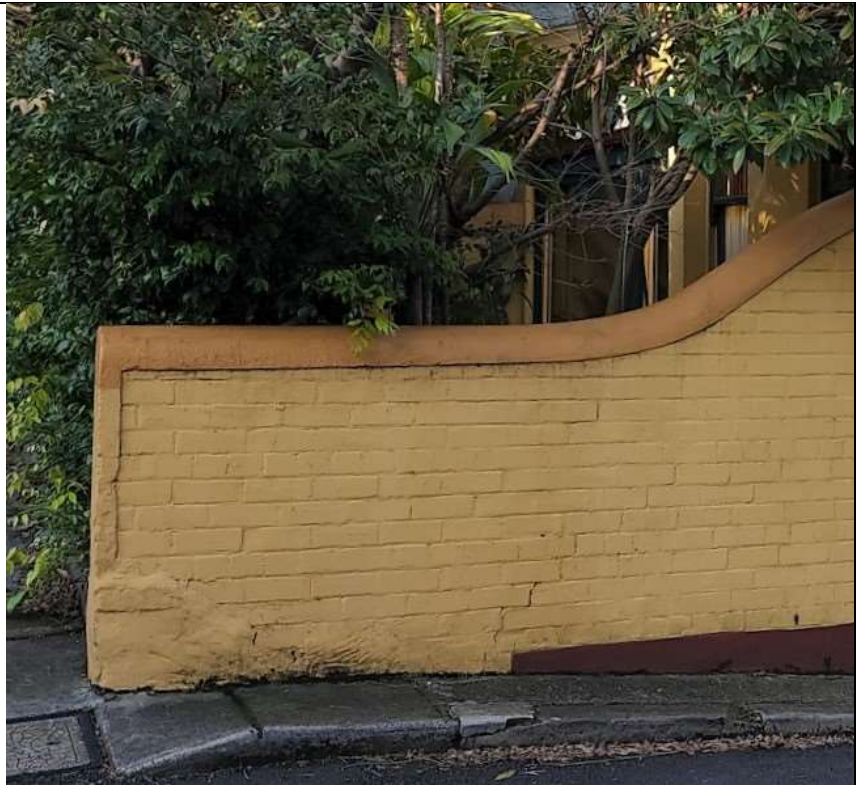
Figure 7 Another example of the way height transitions were managed on traditional fences in the Toxteth Heritage Conservation Area
