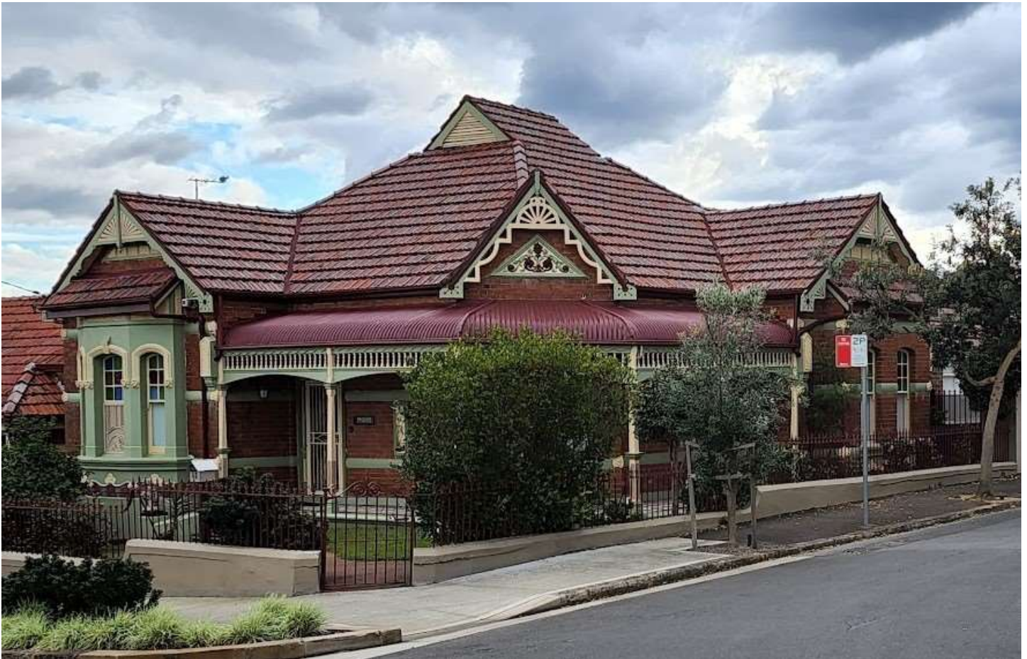
Fig 1 The house exhibits considerable panache in the way it addresses the corner block. It has three gables, one on the SW corner facing Toxteth Road, one on the diagonal facing the corner of Toxteth Road and Maxwell Road and one facing east on Maxwell Road. The front gate is set at the diagonal emphasising that this house has a frontage to two streets.
