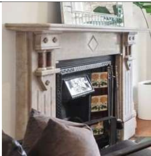
Figure 4 Marble chimney pieces
