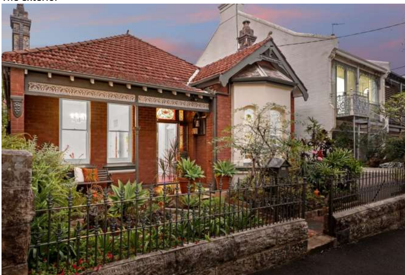
Figure 11 The front of the house
