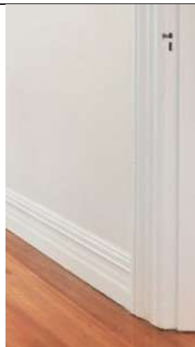
Figure 5 skirting boards and architraves
