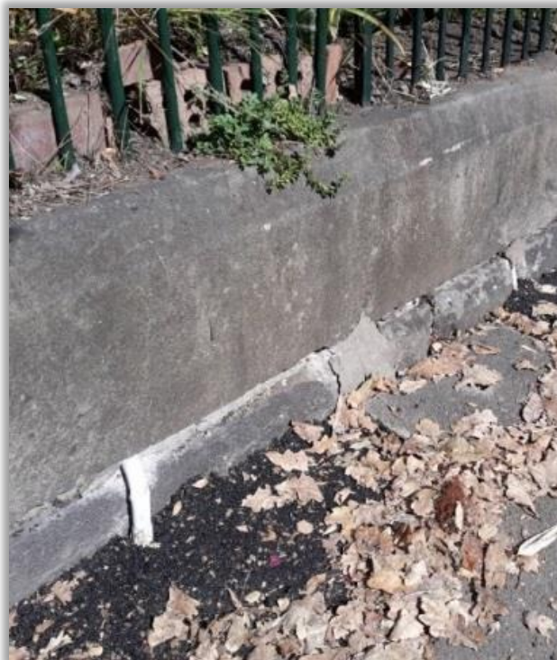
See what NBN contractors can do if they try! Third time lucky – compare this picture to those on the front of last month's Bulletin. The conduit to No. 222 Bridge Rd looks much better while the conduit to No. 224 has been routed through the mortar, and is hardly visible. Surely we can expect at least this level of workmanship throughout our heritage suburb? (image: Olivia Moore)
