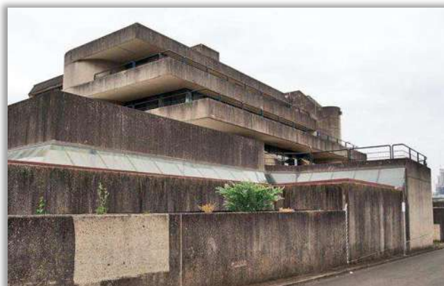
Bidura Children's Court (photo: Jenna Reed Burns http://docomomoaustralia.com.au/ )
