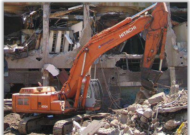
The demolition of the Cowper St public housing complex (image: http://www.aver.com.au/ )
