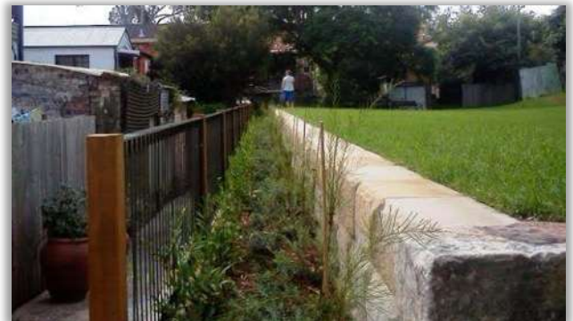
The thriving native flora planted along the new retaining wall in John Street Reserve (image: Friends of John Street Reserve Inc).
