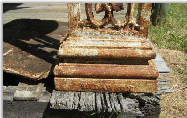
Richard Dawson's own Hebe Cottage at Schofields that still stands in very poor repair. Note the maker's mark at the very bottom of the plate column. (Image Harry Irwin).
