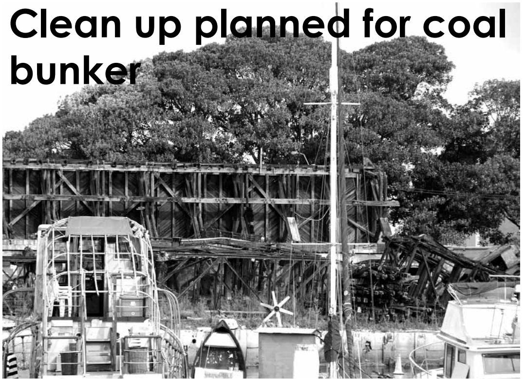
The old coal bunker viewed from the Fish Market. Parts of the dismantled gantry crane can be seen lying in front of the remaining timber structure. Photo: Bruce Davis
