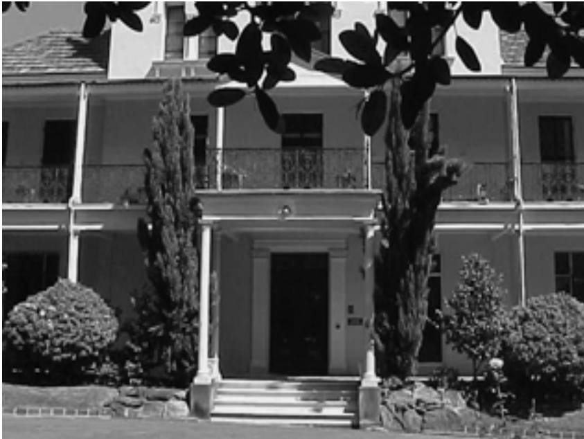
Toxteth House verandah
